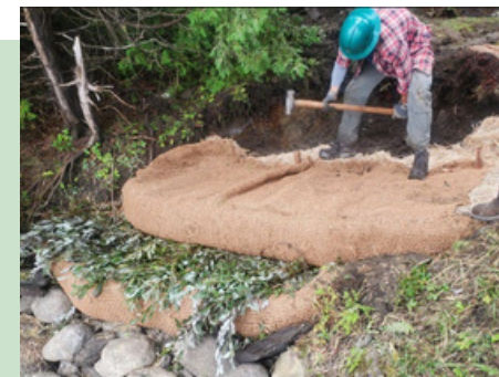
Encapsulated soil lifts installation Caspian Lake, 2023
